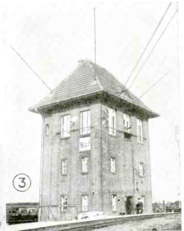
1. Top left—Shows loudspeaker installed in the switch-tower; a two-way conversation is afforded between the tower and the locomotive engineer. 2. Left—shows ultra short-wave phone apparatus installed in a switch tower with train being shunted. 3. Above—One of the switch towers of the Reich railway, showing the antenna masts for the short-wave two-way phone system. 4. Lower left—Engineer with microphone and also loudspeaker in engine cab. 5. Below—Shows box in engine cab containing the whole ultra short-wave transmitter and receiver.
